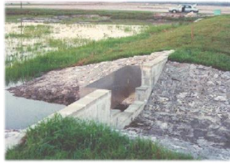
"Wet" Detention Ponds
